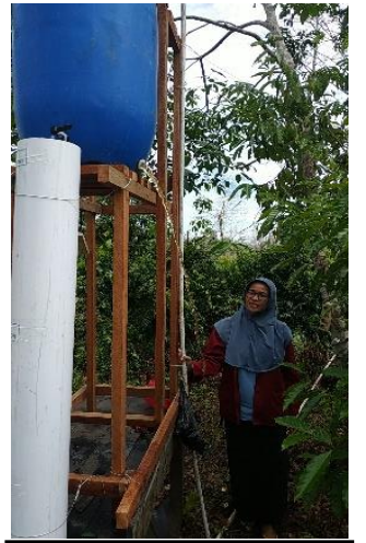
Back Wash Bak 2
